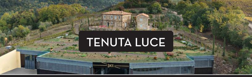
(Pictured) The unique cellar of Tenuta Luce was constructed within a hillside subterranean level, preserving the estate's centuries-old farmhouses above.
